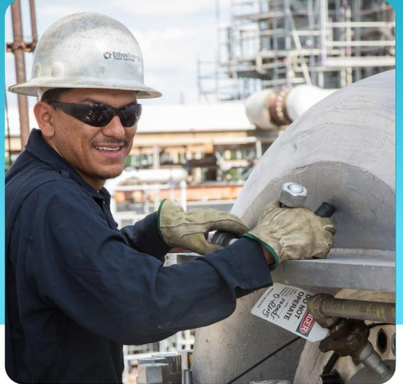
Major overhaul of a TG16 gas turbine in the Tunisian desert. Life extension delivered despite challenging conditions.
